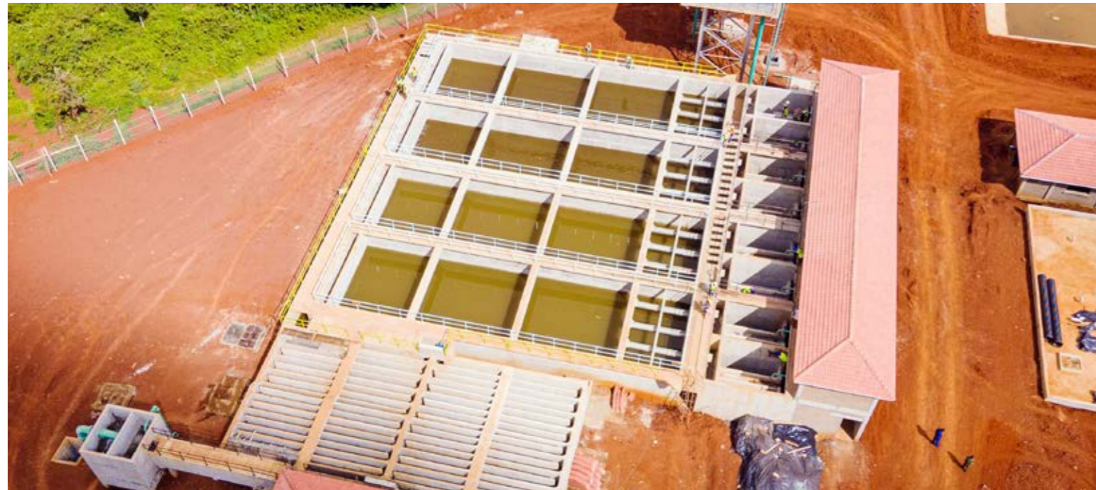
Chuka Water Supply Project - Kirege Treatment Works (under construction).
