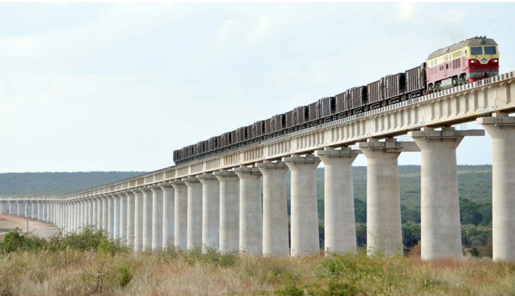
Engineering marvel: A locomotive tests a section of the newly constructed Standard Gauge Railway at Tsavo.
